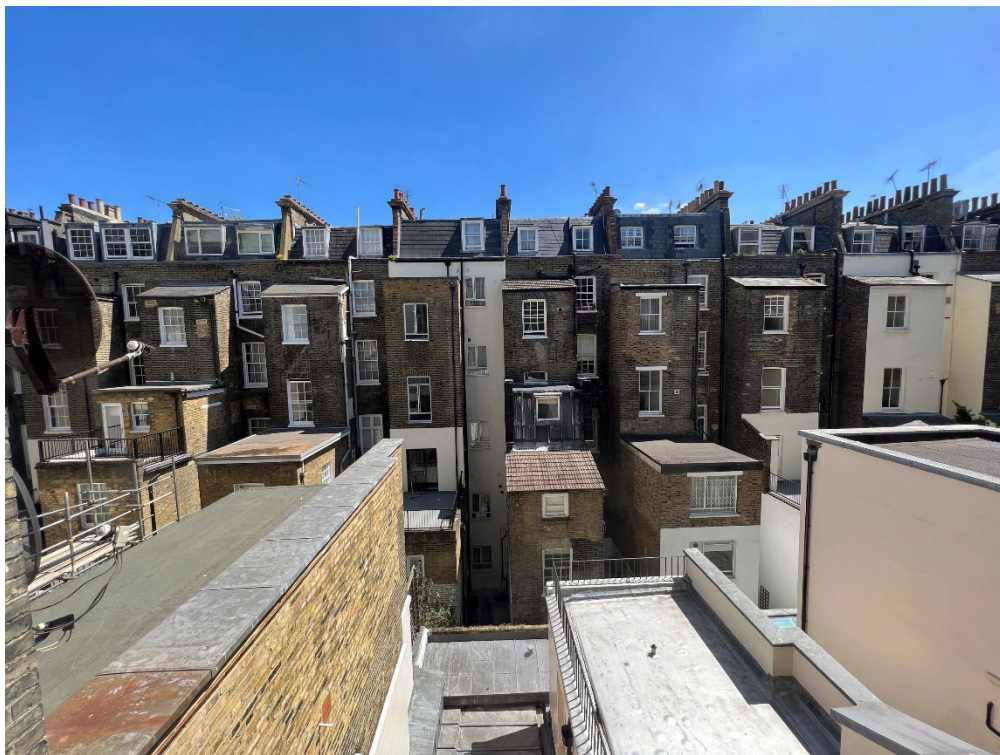
View from the rear of 54 Warwick Square
